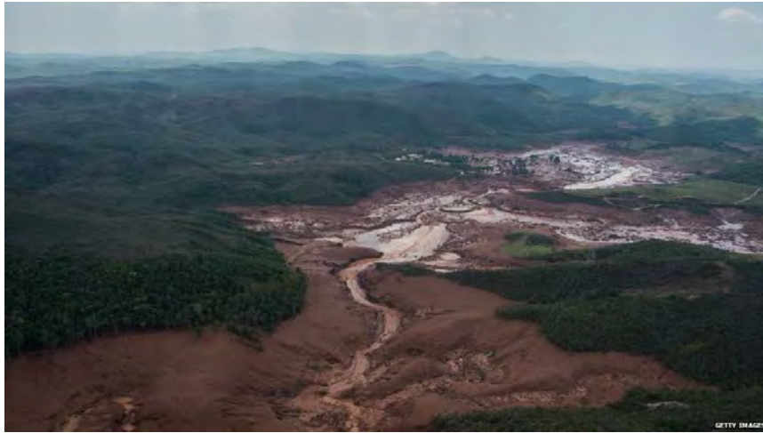
Figure 1: Tailings dam spill in Brazil, 2015. (Getty Images)
